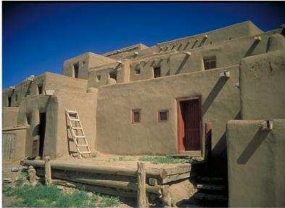
Taos (Pueblo) house, courtesy bradknapp.com
